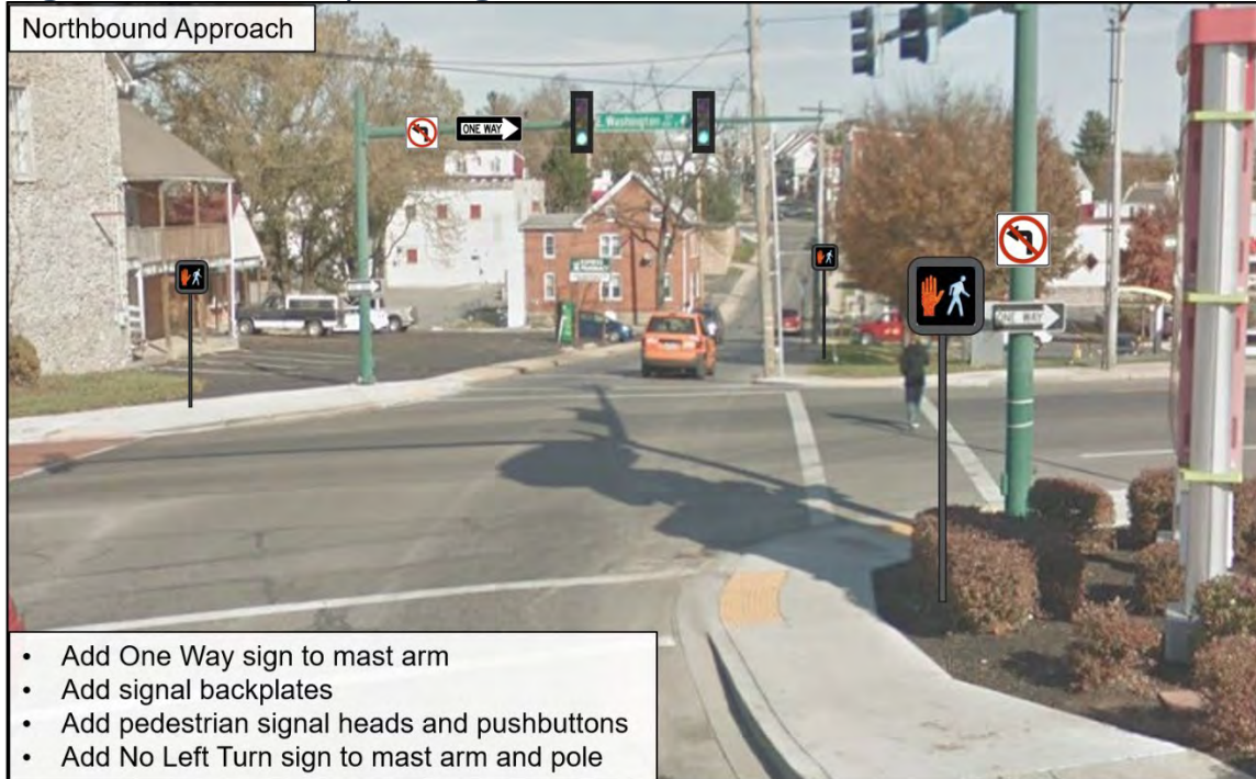
Figure 32: Cannon Ave/Washington St Intersection – Northbound Recommendations
